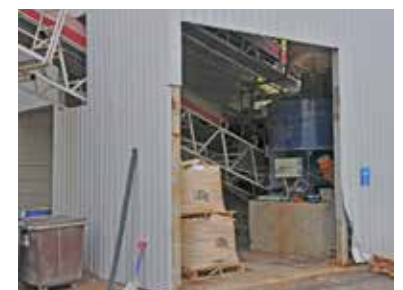
Installation example of 2 pcs MD500 in Japan. Dual dosing equipment for optimisation of steel fibre concrete production for flooring and shotcrete.
